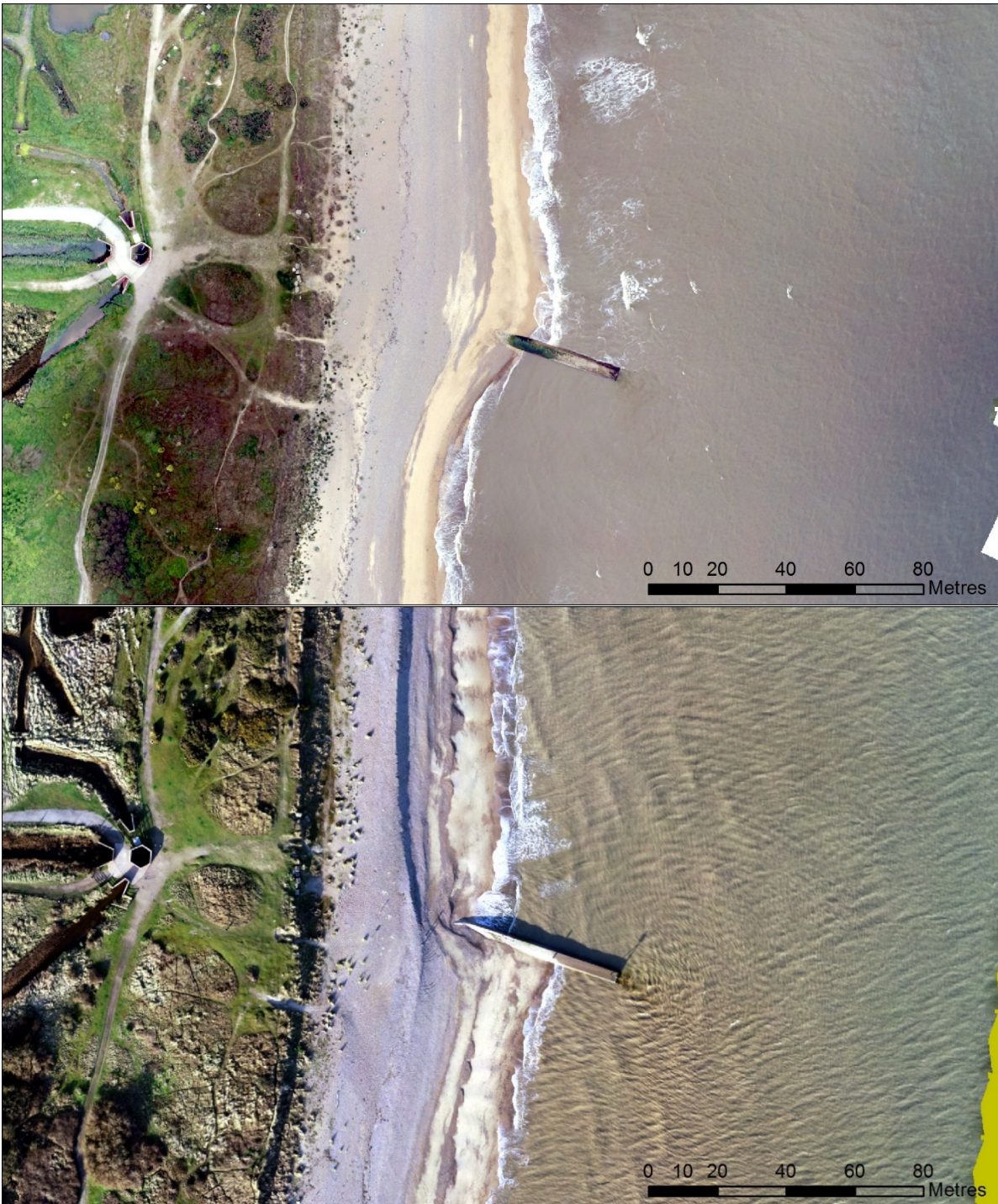
Figure 2: Downtide erosion and updrift accretion resulting from the partial blockage to longshore sediment transport caused by the Minsmere Sluice Outfall following NE (top) and SSE (bottom) storm conditions.
